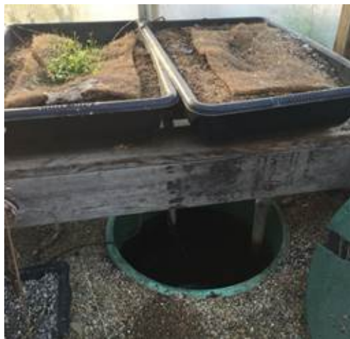
Figure 9: System Midpoint sampling location.
