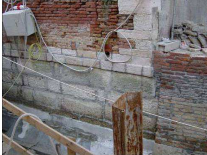
Figure 4: Canal Wall Undergoing Repair 4
