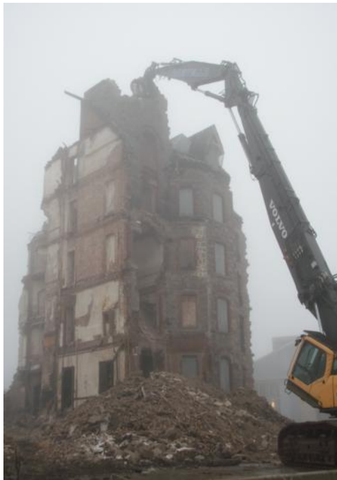
Figure 3: Costello dismantling the Clock Tower
