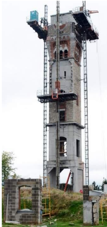
Figure 5: Gilbane's progress of Construction on the Tower
