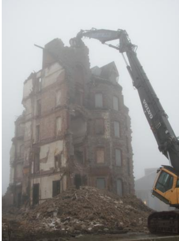
Figure 3: Costello dismantling the Clock Tower
