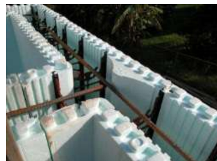
Figure 19: ICF Interlocking Form (Walls)
