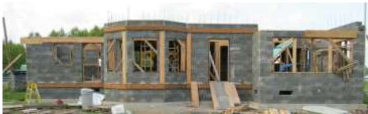
Figure 30: FasWall Project in Progress (FasWall Home)
