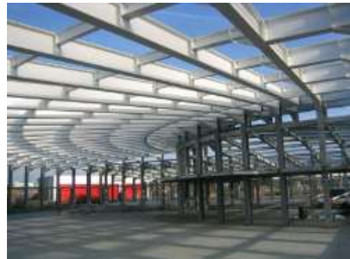
Figure 21: Structural Steel (Services)
