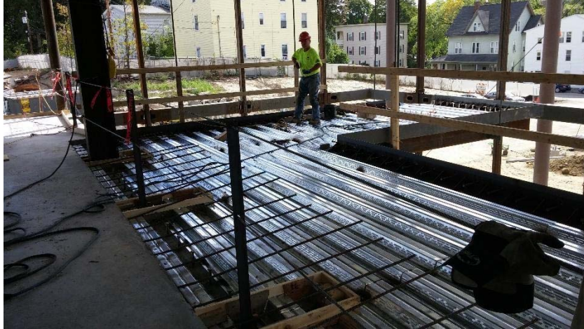
Figure 1 Slab-on-metal decking in the ASEC
