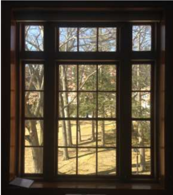
Figure 8 Existing windows installed in Kaven Hall
