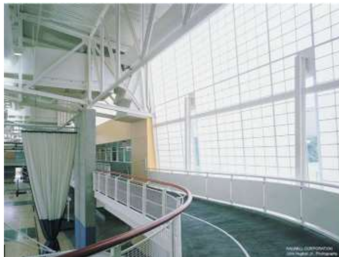
Figure 10 example of translucent aerogel insulation as a high performance thermal insulation solution for daylighting [31]
