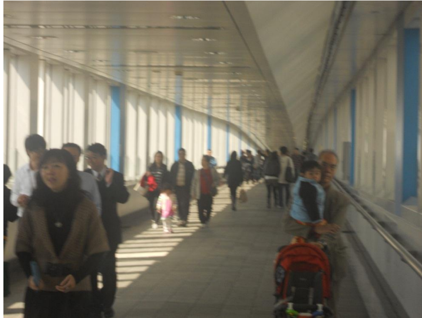
Figure 5.1-4 MTR Exit E Footbridge
