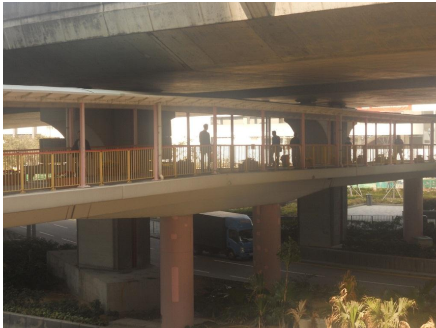
Figure 4.4-20 - Footbridge to Sun Yat Sin Park in Sai Ying Pun
