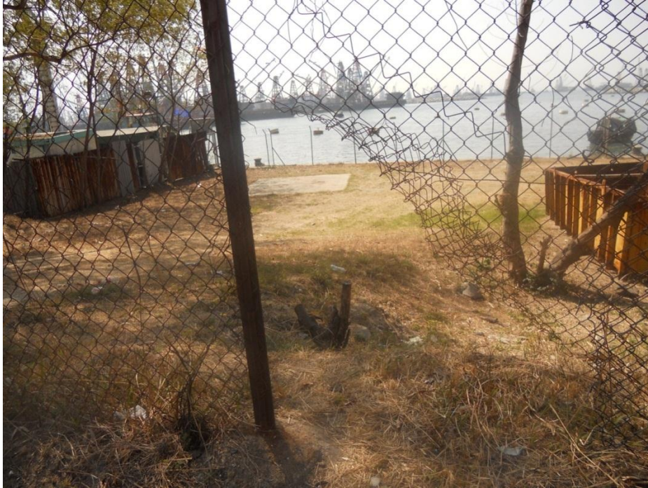
Figure 5.1-3 Hole in Fence for Waterfront Access
