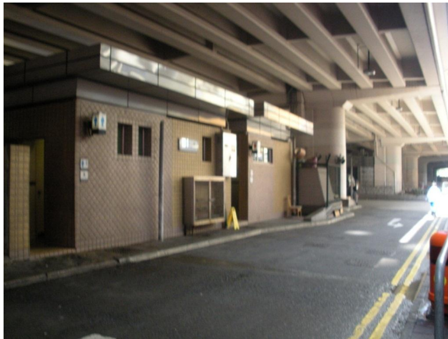
Figure 5.1-11 - Poor Aesthetics along Route in Wan Chai
