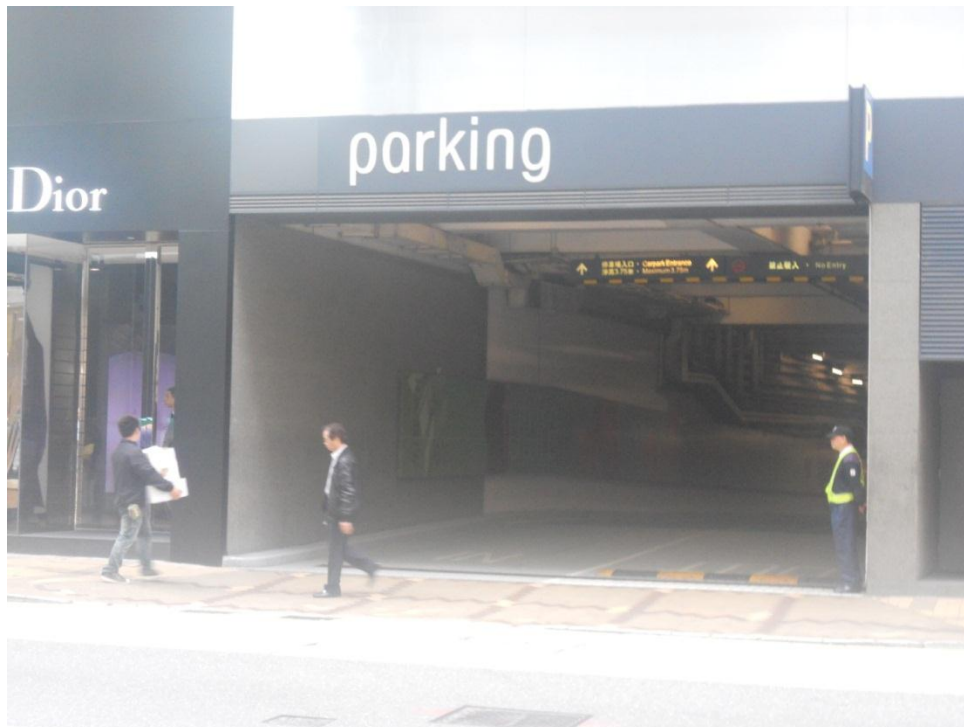
Figure 5.1-5 Parking Garage on Canton Road
