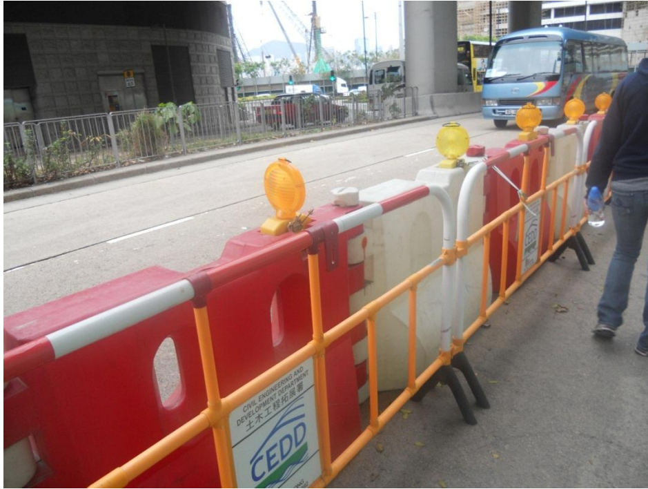
Figure 5.1-7 Construction Detour on Chatham Road South
