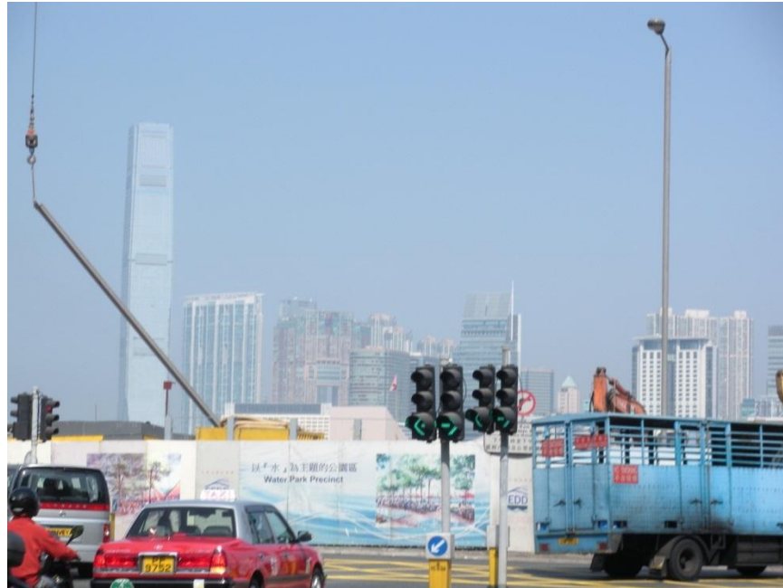
Figure 5.1-10 - Construction Breakdown Point in Wan Chai
