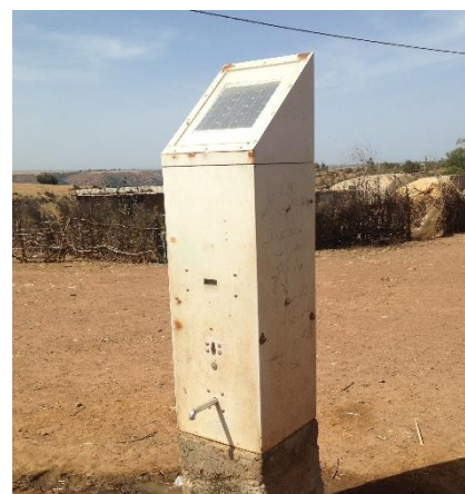
Figure 2: A solar powered, coin-operated water pump that pumps water from a well to provide drinking water for community members
