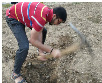
Figure 11: Abhay digging the foundation for the nursery prototype
