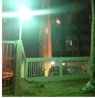
Figure 22: Luminaire in Quadrant 9
