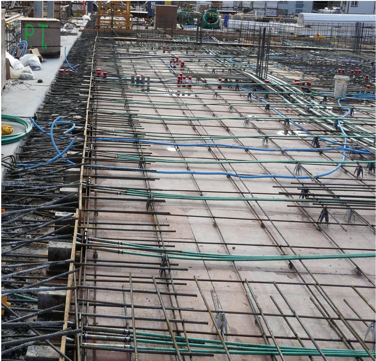
Figure 2: Post tensioning cables laid before a concrete pour
