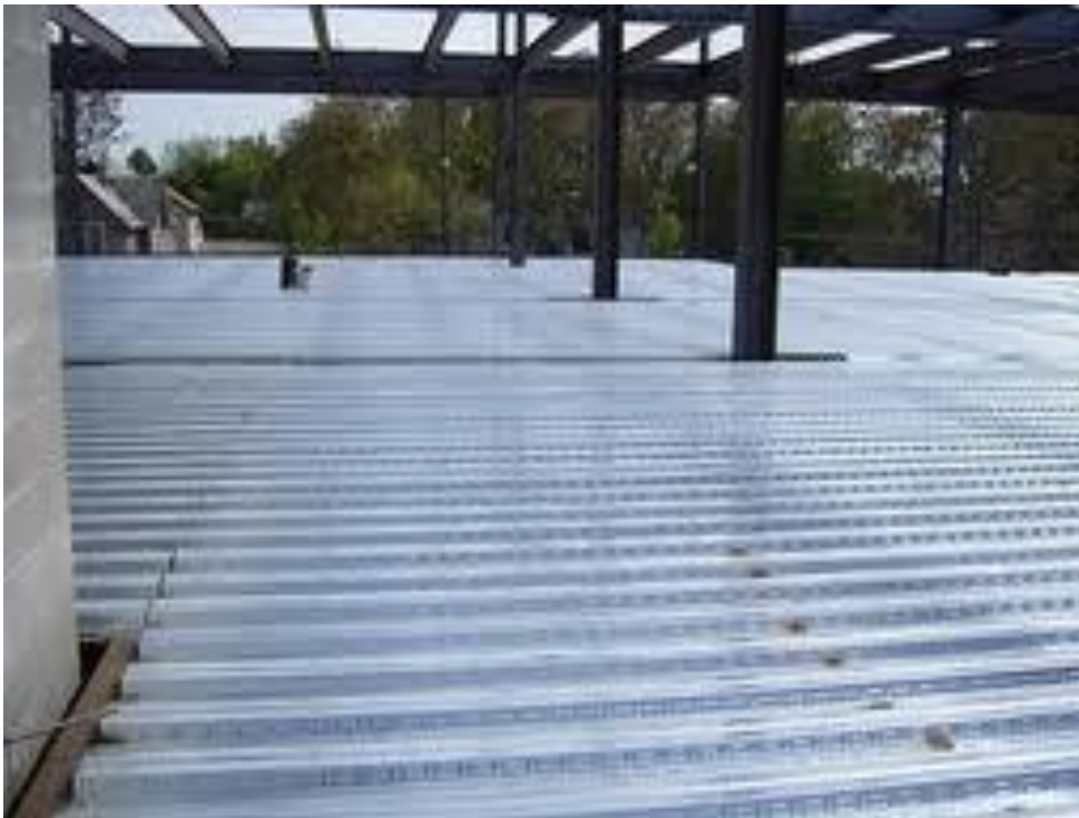
Figure 7: Steel decking before a concrete pour 5
