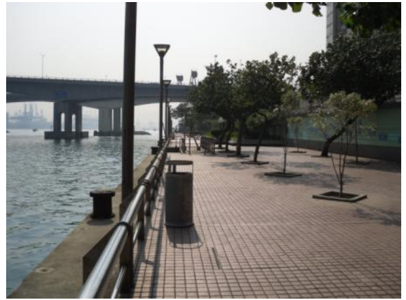
26 – Cheung Fai Road Promenade (1)
