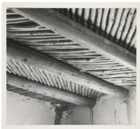
Figure 4 - Vigas and Latillas (Adams, 2018)
