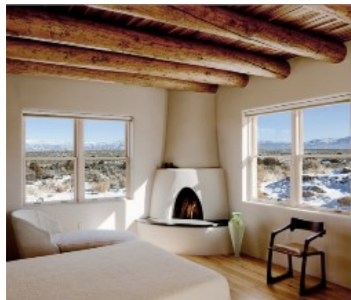
Figure 7 - Interior Example of Contemporary Puebloan Architecture with Visible Vigas and Latillas (Gittings, 2012)
