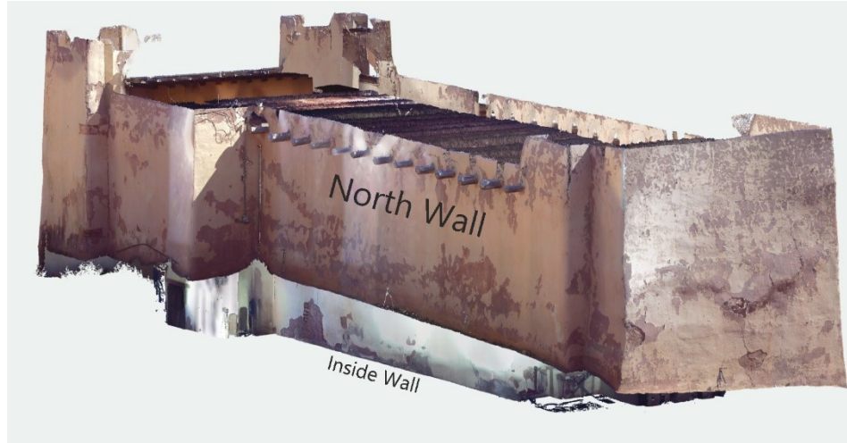
Figure 14: Obscured North wall LiDAR Data
