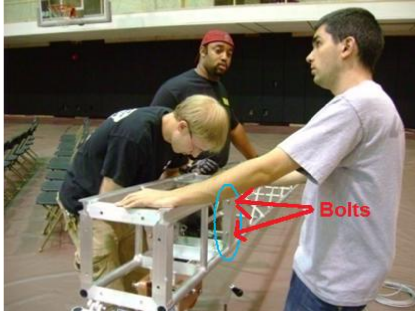
Figure 12: Bolting the tower truss onto the unhinged tower
