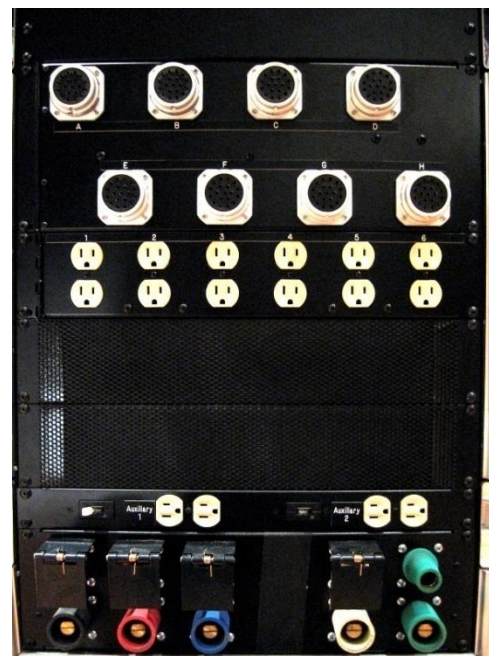
Figure 2 - Rear of a typical dimmer rack.
