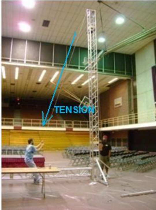
Figure 16: Tension is applied to the aircraft cable as it is cranked
