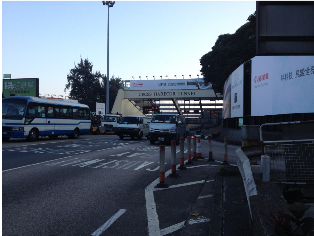
Figure 32: Exiting lane to Causeway Bay of the Cross-Harbour Tunnel (Courtesy of Adria Fung)
