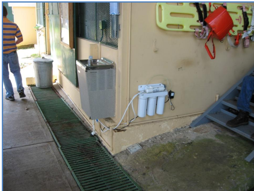
Figure B-2: Filter for Water Fountain at Dock
