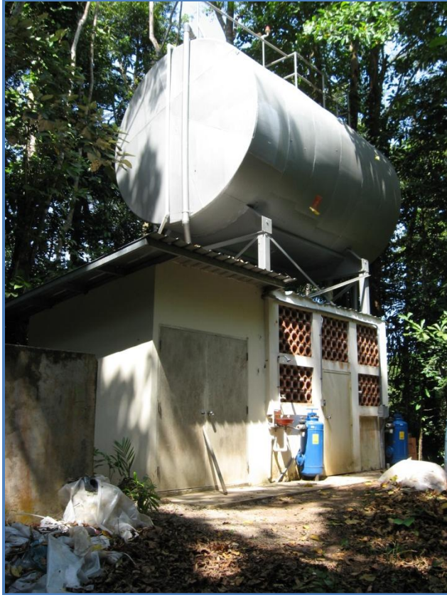
Figure A-11: 16,000 Gallon Metal Tank on Top of Filter Shed
