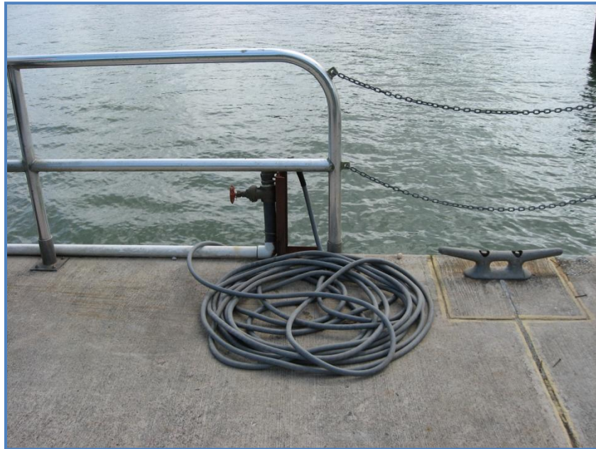
Figure C-1: Potable Water Line Extended from ACP Dredging Division, Jan. 13, 2010
