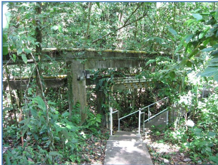
Figure A-12: Pipeline Leading to the Distribution System for STRI
