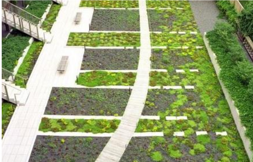
Figure 55: Extensive green roof on 29 Garden St, Harvard University, Cambridge, MA
