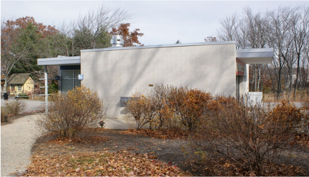
Figure 3. Southwest Facing Wall
