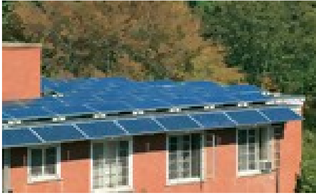
Figure 4. Canter levered Modules
