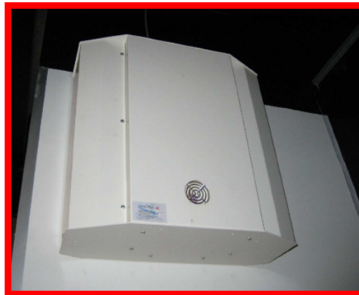
Photo 2 = Smoke generating unit
