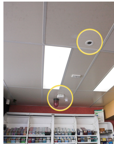
Fig. 4.5.2B – Ceiling Nozzle and Feedback Sensor
