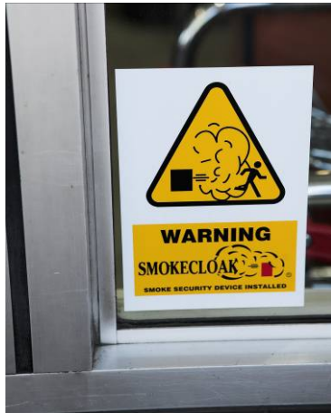
Fig. 4.5.4E – Warning Signage on Front Window
