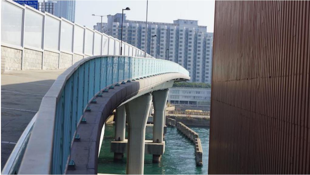
FIGURE 17: THE HUNG HOM OVERPASS CONNECTING THE TST EAST PROMENADE AND THE HUNG HOM PROMENADE. (COURTESY OF BETH LACARRA, 2014)
