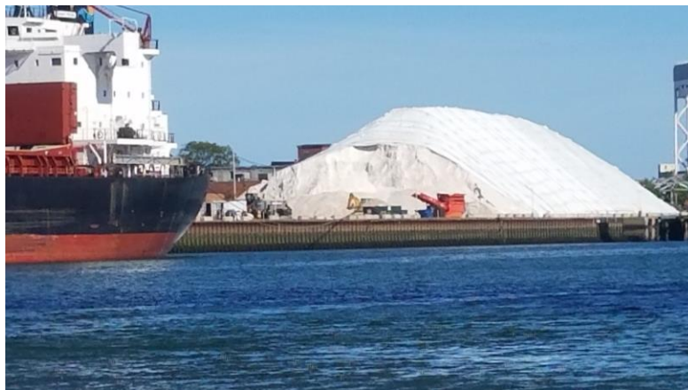
Figure 10: Bulkhead located at Eastern Salt
