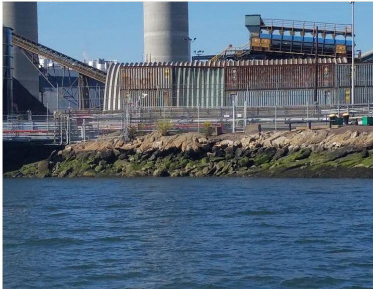
Figure 9: Riprap located at Prolerized
