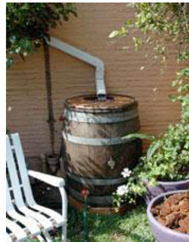
FIGURE 14: BARREL STORAGE TANK (CITY OF PORTLAND, OR)
