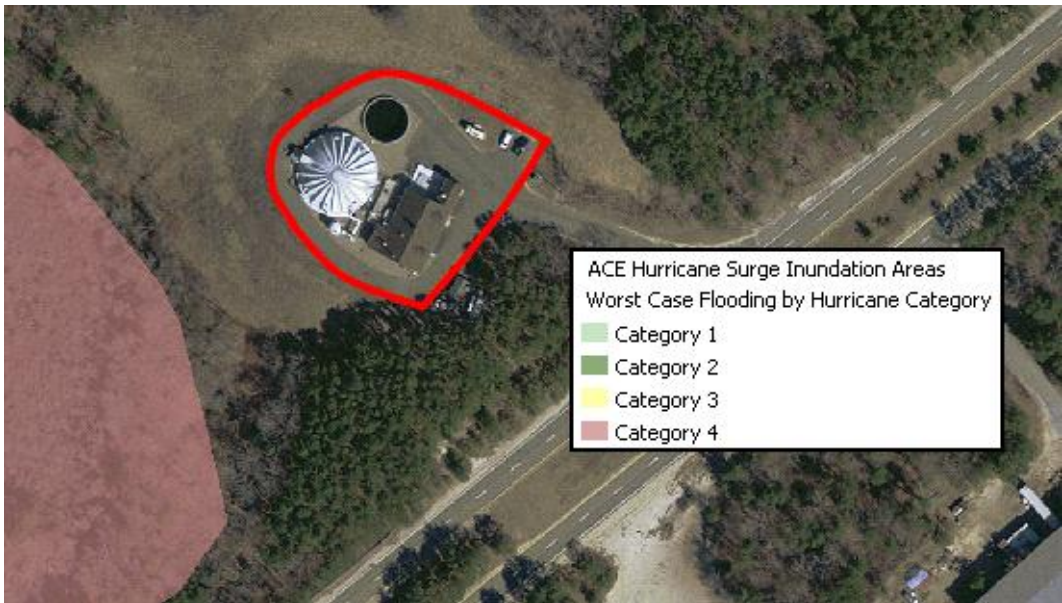
Figure 5. 4: ACE Hurricane Inundation Area map for the Provincetown Wastewater Treatment Plant
