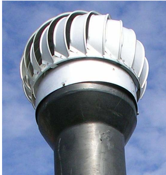
Figure 4.5: Whirlybird mechanism used for ventilation of the Enviro Loo.
