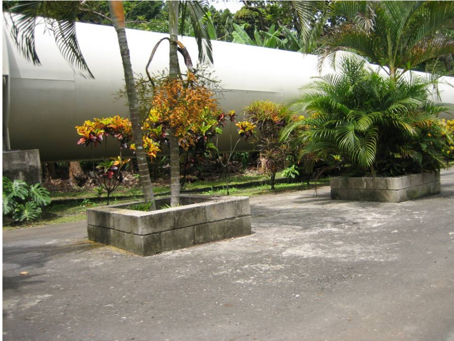
Figure 18: Aqueduct Used to Transport Water to the Turbine
