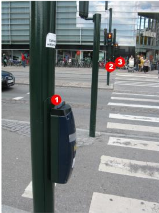
Figure 17: All APS devices are along the same side of the crosswalk.
