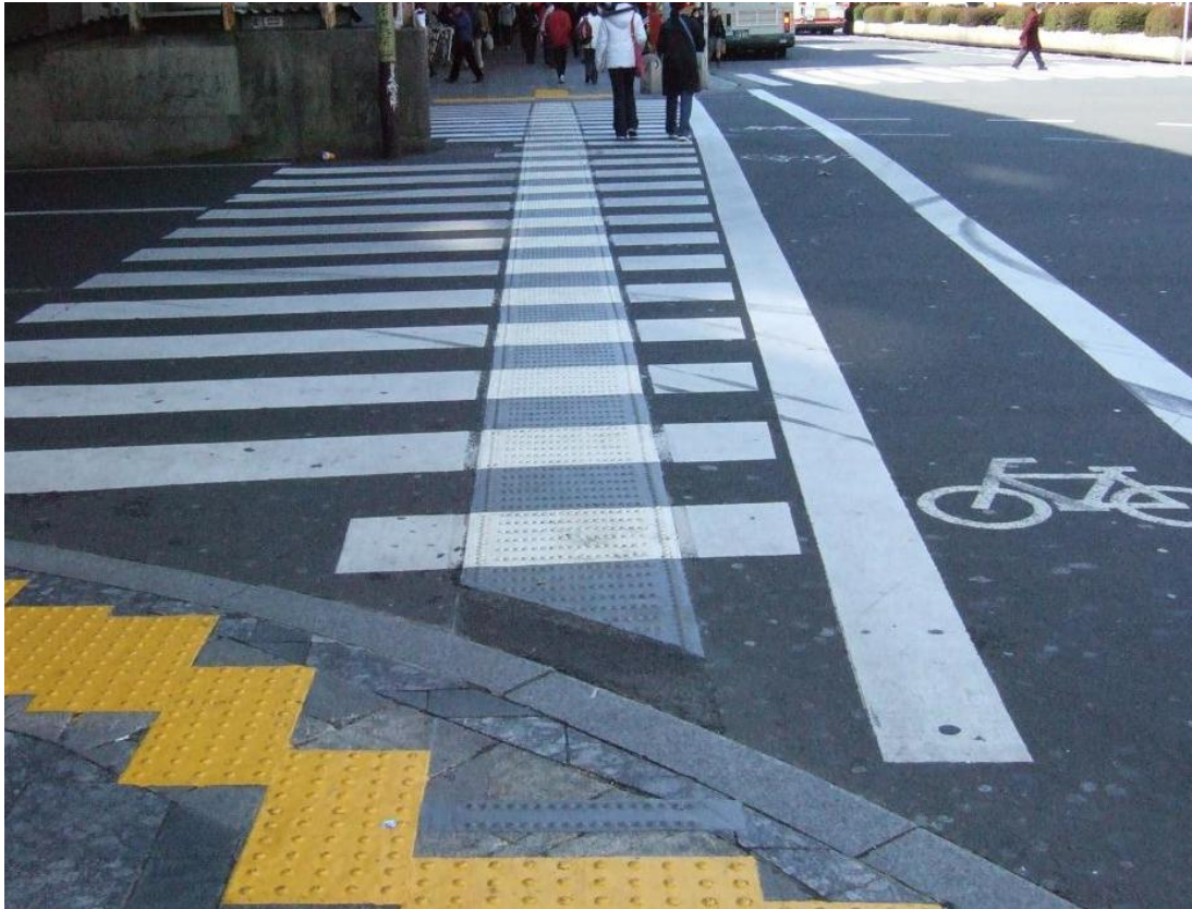
Figure 11: Tactile path crossing a street in Japan (“Tactile Guiding Line”, 2006)
