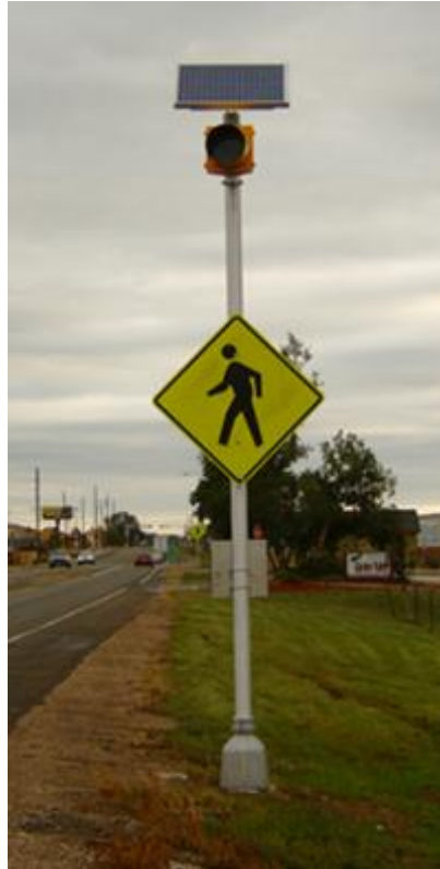
Figure 25: Wireless pedestrian warning sign (Northwest Power Co., 2010)
