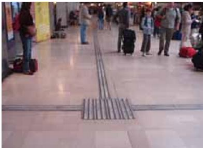
Figure 9: Directional blocks forming tactile path in France (Katsumi et al., 2008 9)
