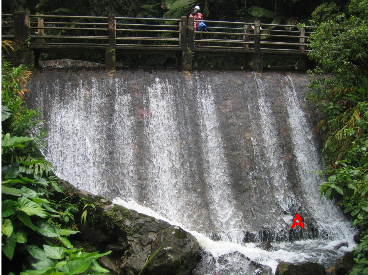
Figure 4.8: Baño Grande Dam at the Palo Colorado Recreation Area
