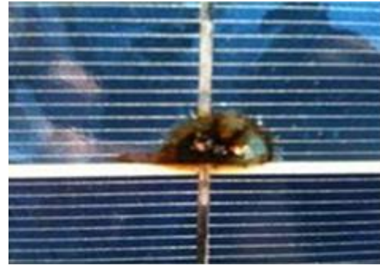
Figure 9: Module hot spot failure (First Green, 2014)
