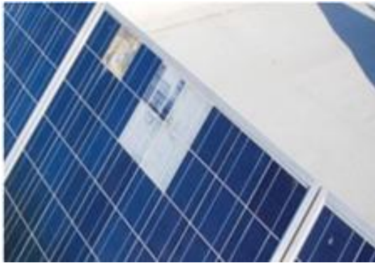
Figure 8: Module delamination failure (First Green, 2014)
