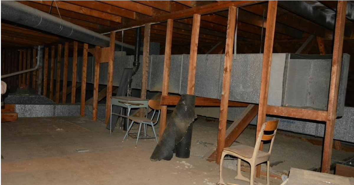
Figure 25: The Unfinished Section of the Attic, Ideal for Senior Center Seasonal Storage
