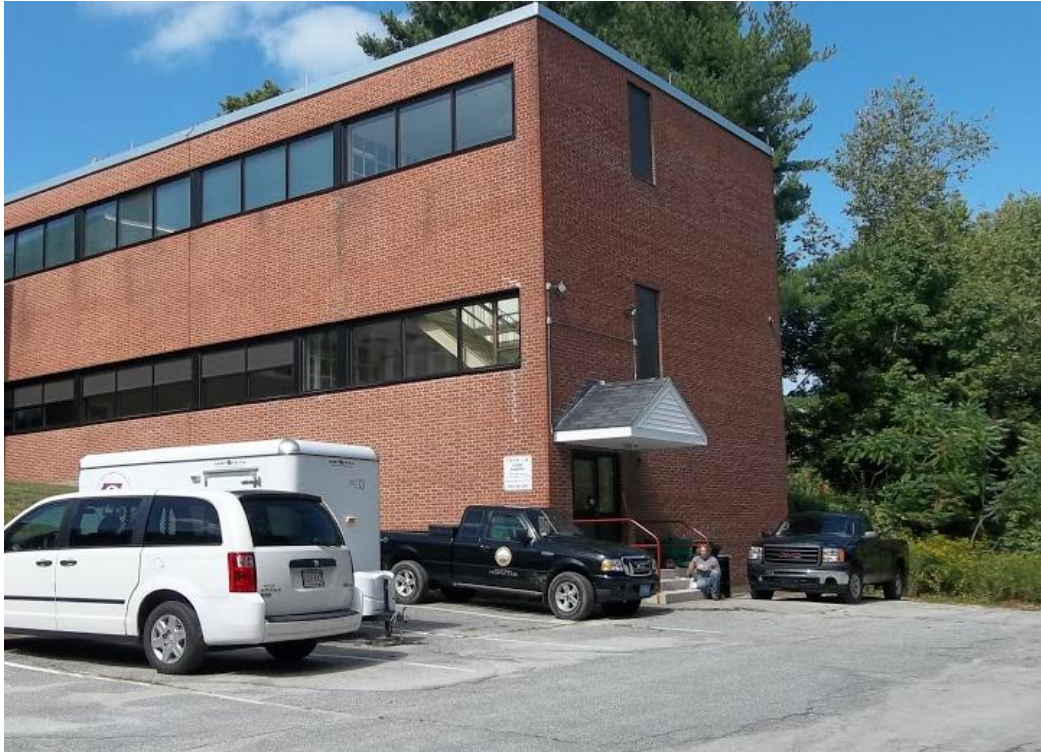
Figure 27: The Door by CHIP-IN is Non-compliant
