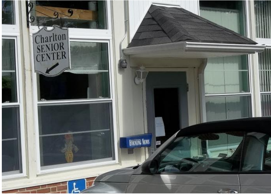
Figure 18: The Exterior Senior Center Door with Obstructing Mailbox
