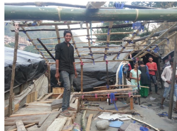
Figure 13. School under construction
