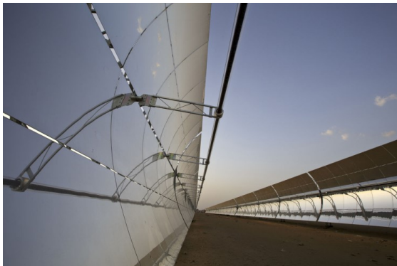
Figure 2. Parabolic mirrors focus the sun at a 50 MW CSP installation in Rajasthan, India (Pearson, 2013)
