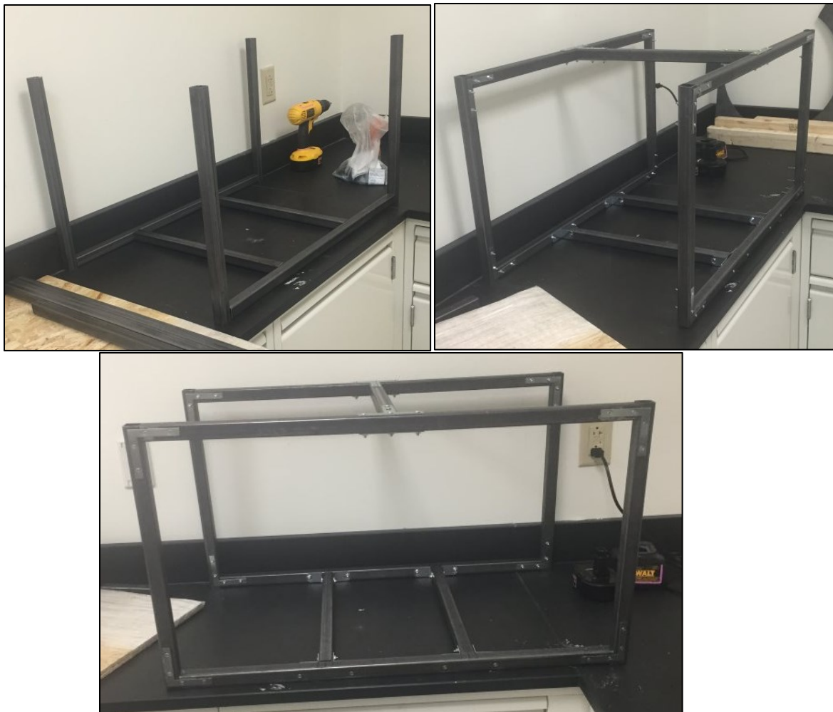
Figure 24 Assembly of the Frame
