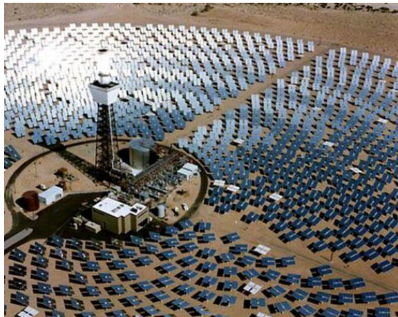
Figure 15: Large Solar Array Located in a Desert (Ecofriend, 2008)
