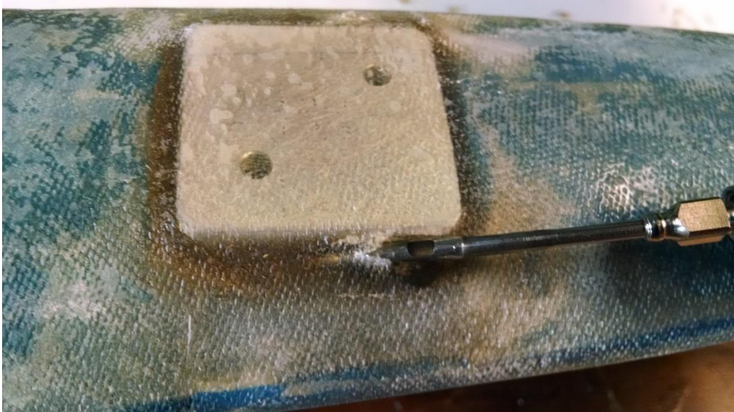
Figure 38 - Basting needle injecting epoxy resin into gap between fiberglass, plate, and hull
