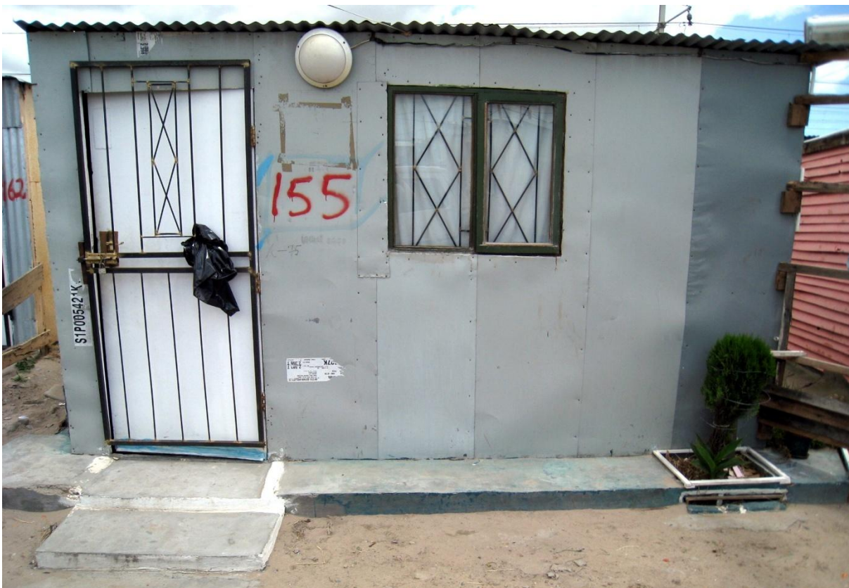
Figure 19: Use of concrete flooring in Lotus River to reduce seepage
