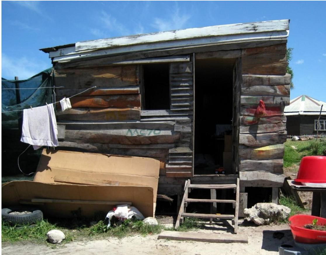
Figure 20: Use of stilts in Marcus Garvey to prevent seepage
