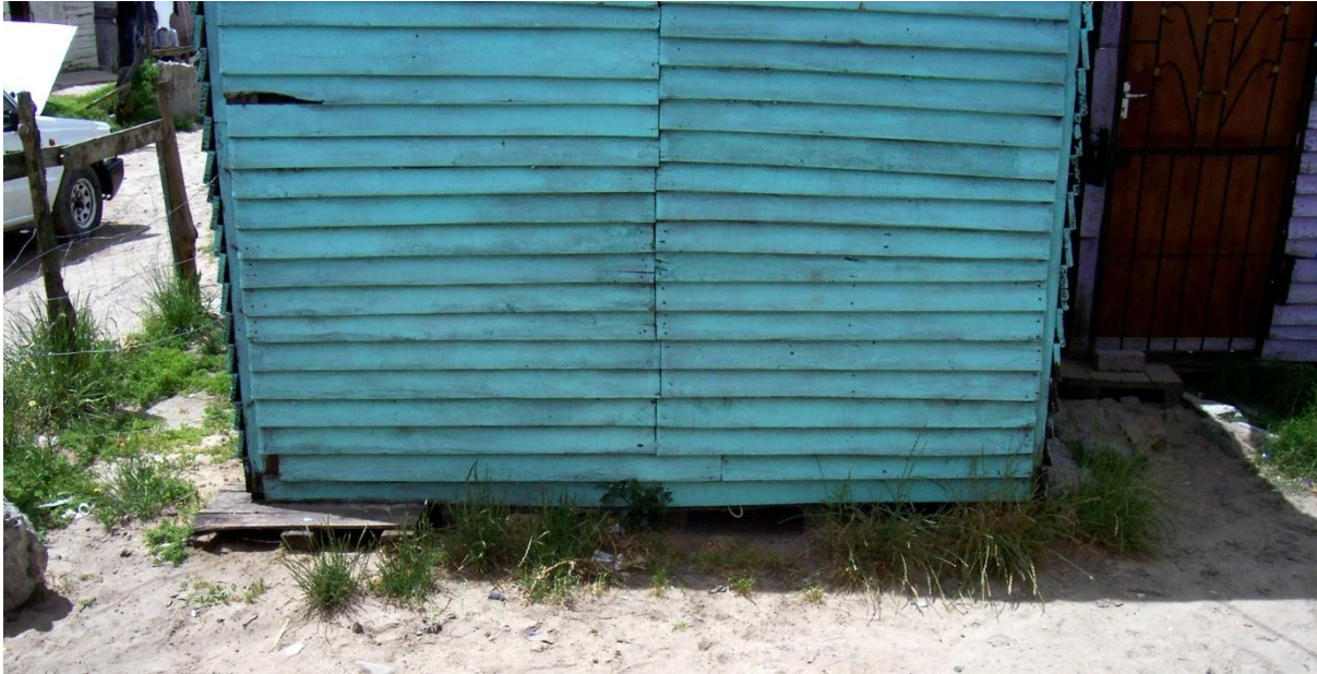
Figure 18: Use of pallets in Lotus River to prevent seepage
