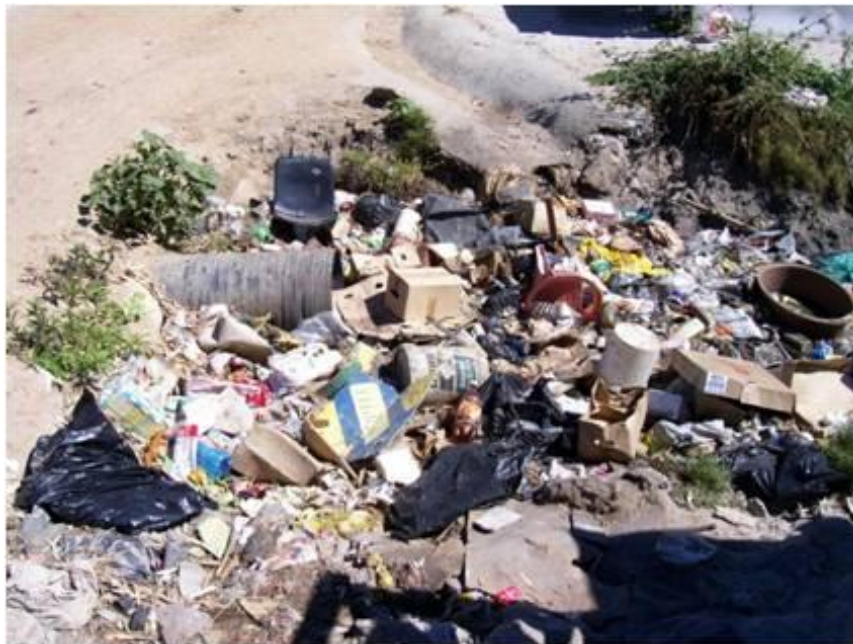
Figure 22: Blocked infrastructure in Phola Park Philippi
