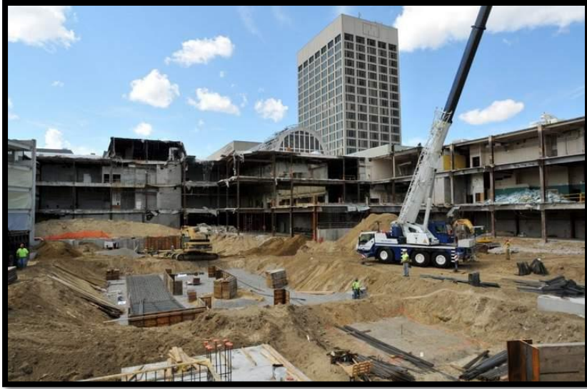
Figure 5 - Demolition of Worcester Commons Fashion Outlets (Grillo, 2013)
