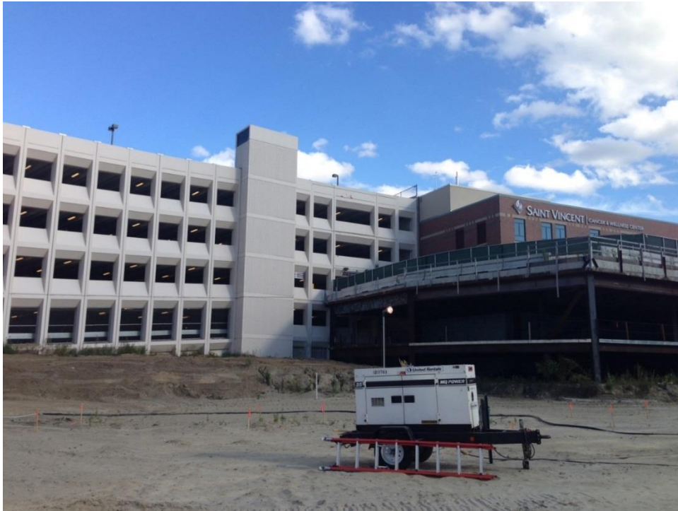
East Garage Mitigation area from Ball field area view
