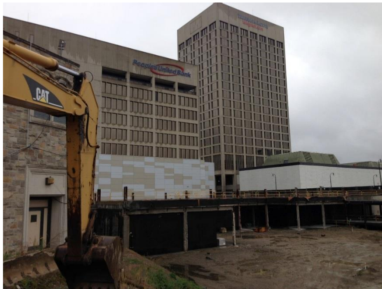
Building E Area from Trumble St. View
