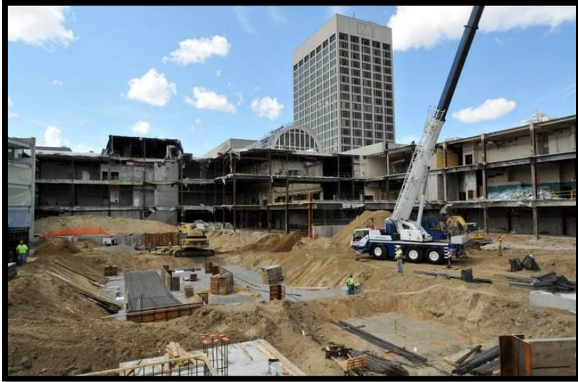
Figure 5 - Demolition of Worcester Commons Fashion Outlets (Grillo, 2013)
