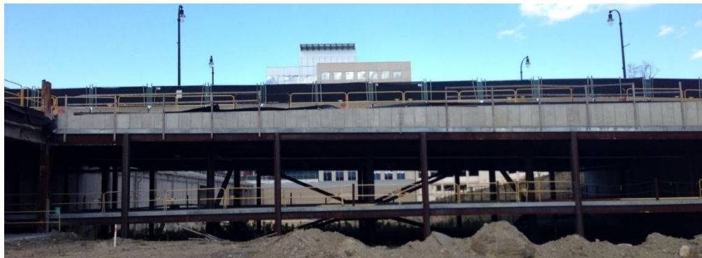
Front St. bridge
