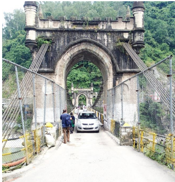
Figure 12: Victoria Bridge – one-way, very slim bridge
