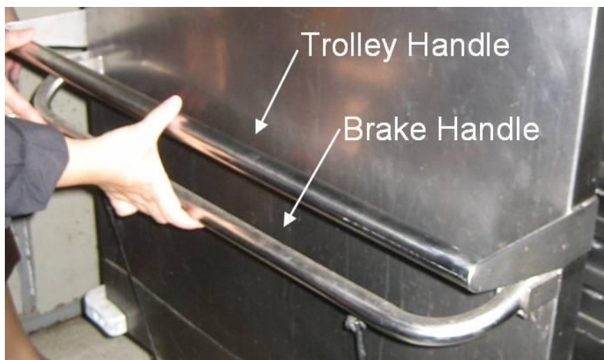
Figure 27: An Operator Using the Current Brake
