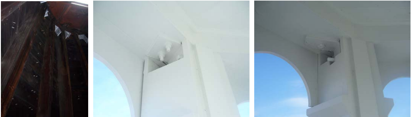
Figure 22: Views of Tower Bracing
