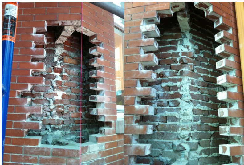
Figure 19: Washburn Tower Masonry Wall Cross-Sections
