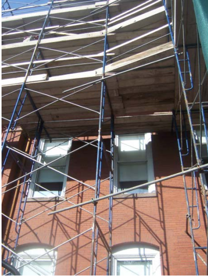
Scaffolding on Front of Building
