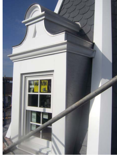
New Window on Tower
