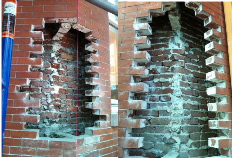
Figure 5. Washburn Tower Masonry Wall Cross-Sections
