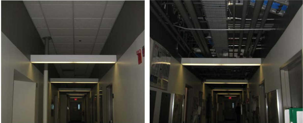
Figure 83: Washburn Ceilings (third floor on left, second floor on right)
