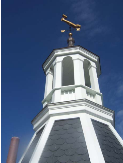
Top of Tower
