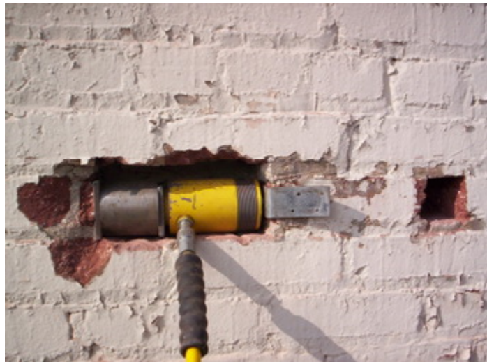
Figure 13. In-place Shear Test
