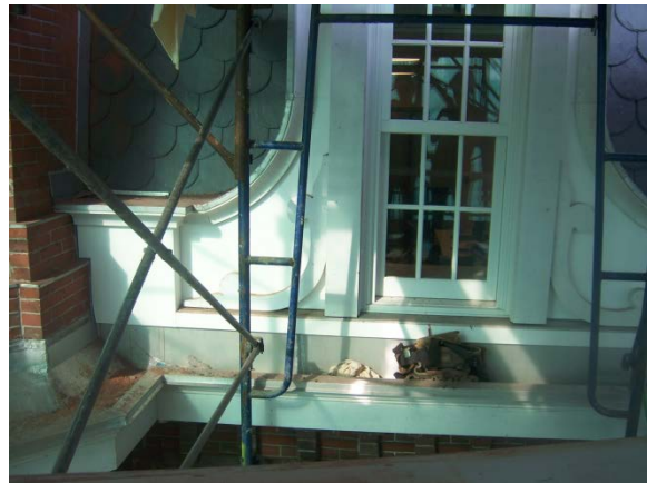
New Window at Roof Level
