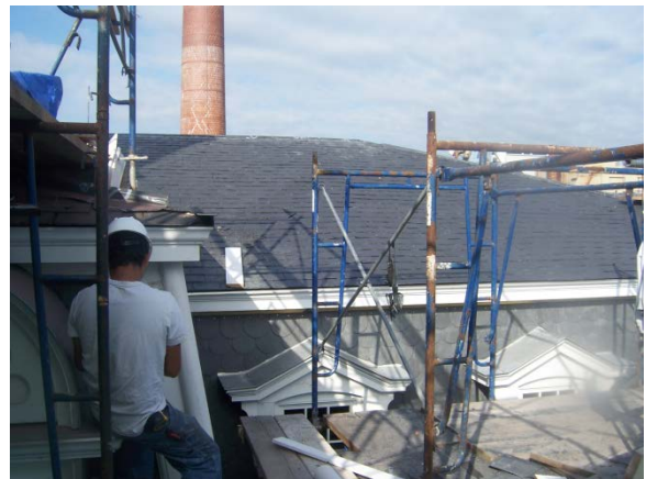
Top Windows and Roof
