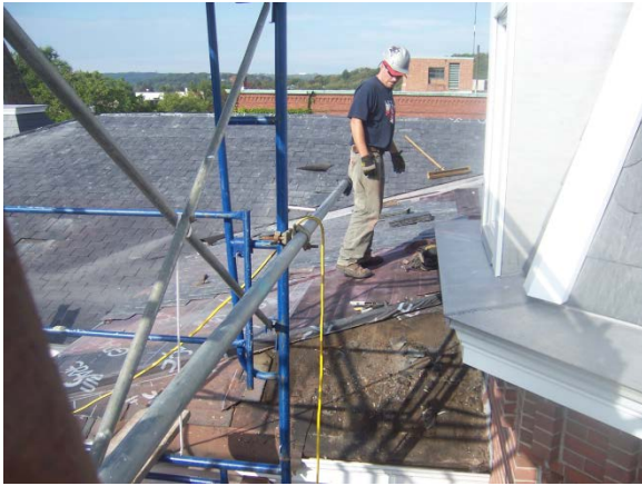
Working on Roofing
