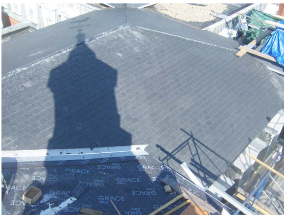
Roof from Top of Tower
