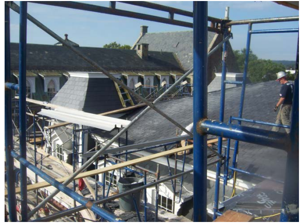
Laying Slate on Roof
