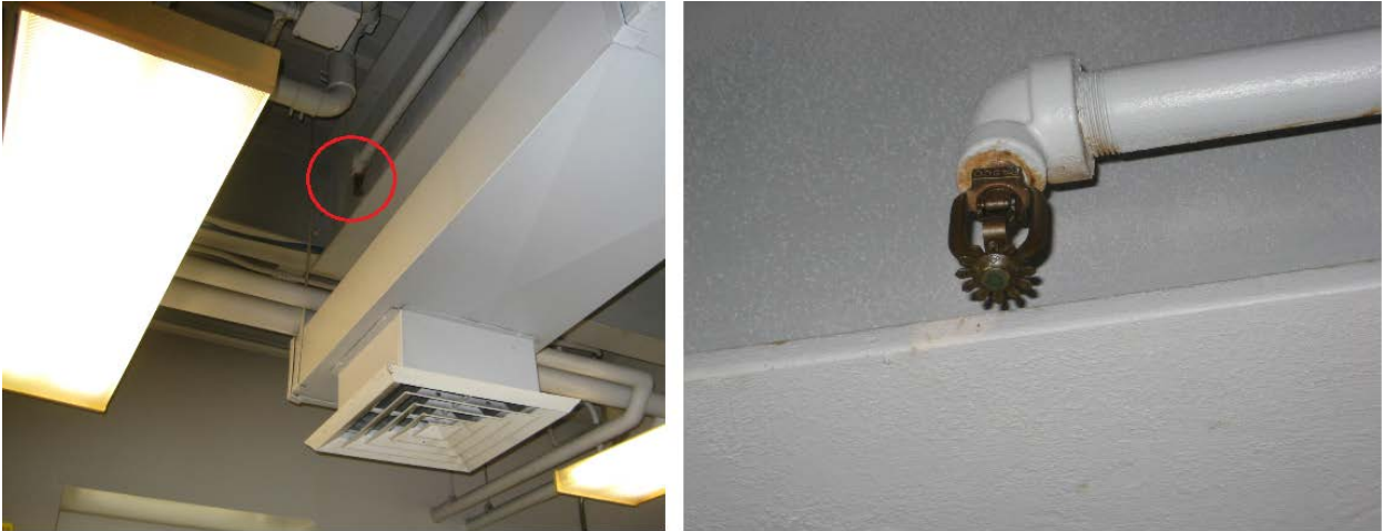
Figure 56: Beam Obstruction Room 339
