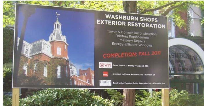
Figure 18: Sign Announcing Renovation
