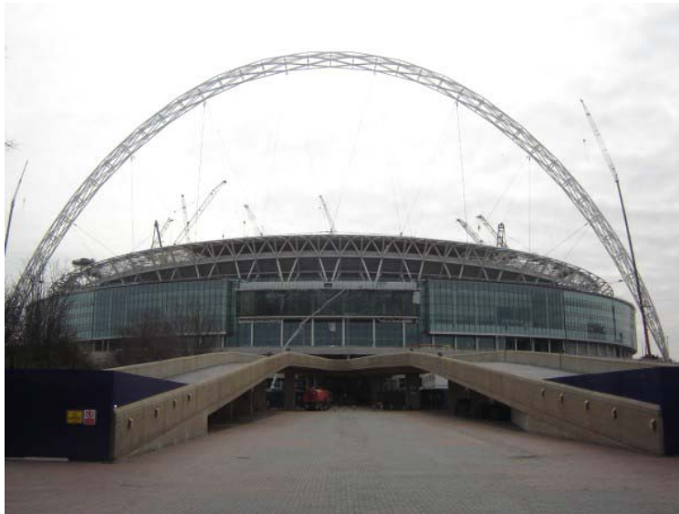
Figure 1: Wembley Stadium March 2006
