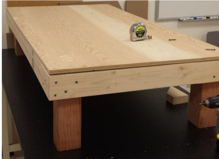
Figure 15: Wood Frame Base with Top Floor Board
