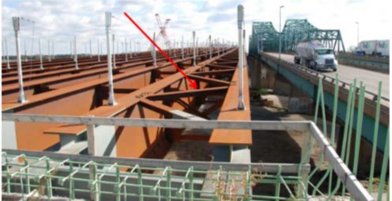
Figure 11: Lateral Bracing (Shaner, J. 2016)
