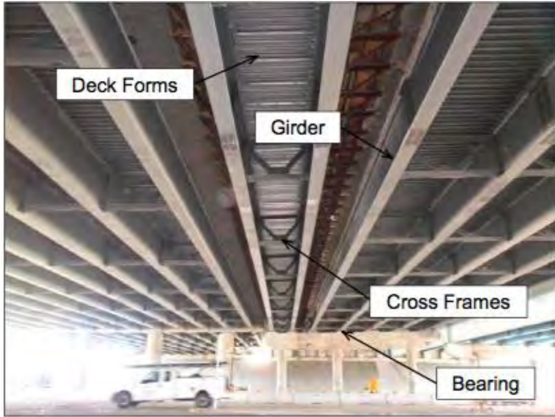
Figure 2 - Bridge Superstructure (Shaner, J. 2016)
