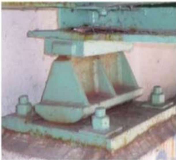
Figure 12:Rocker Bearing (Shaner, J. 2016)
