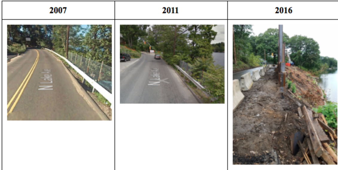
Figure 4: North Lake Ave during 2007, 2011, and 2016 respectively
