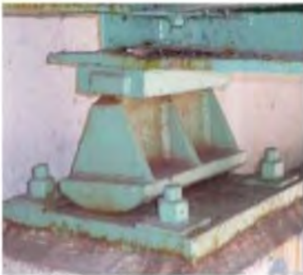
Figure 6 - Rocker Bearing (Shaner, J. 2016)
