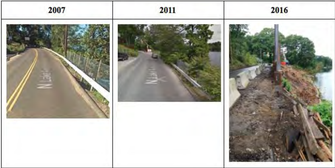
Figure 1 - North Lake Ave during 2007, 2011, and 2016 respectively
