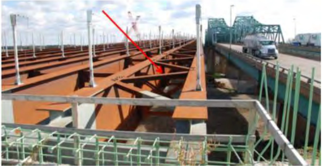
Figure 5 - Lateral Bracing (Shaner, J. 2016)
