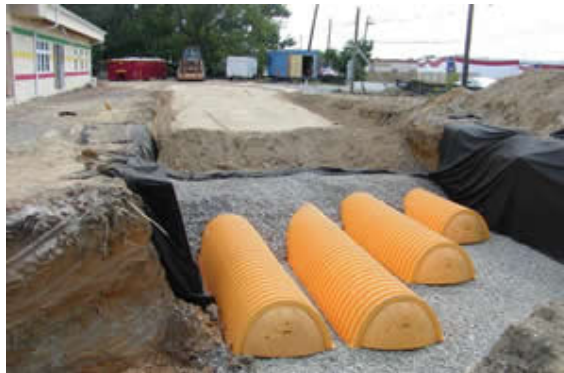
Figure 3-StormTech Chambers (StormTech, StormTech SC-740 Chamber )
