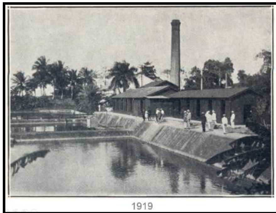
Figure 4. Picture of the site of the Antiguo Acueducto in 1919.
