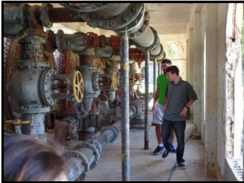
Figure 9. Site of the Antiguo Acueducto. (a) Water filter tank that belongs to the site of the Antiguo Acueducto and was acquired later by Trust after being taken from the site. (b) Current condition of the mechanical water filtration system.
