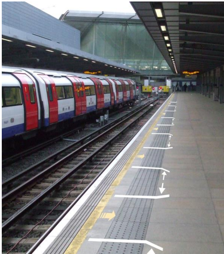
Figure 25. Visualization of Markings demonstrated on the non-PED Jubilee Line platform at Stratford.
