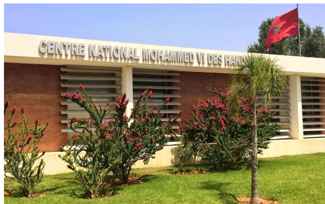
Figure 2.1. Photograph of the Mohammed VI Center for the Disabled in Salé, Morocco (Centre National Mohammed VI des Handicapés website, 2014)
