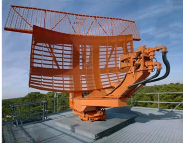
Figure 7: Airport Surveillance Radar. Rotating dish radar with fixed aperture. (Wikipedia)
