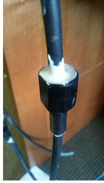
(a) Cables being epoxied
