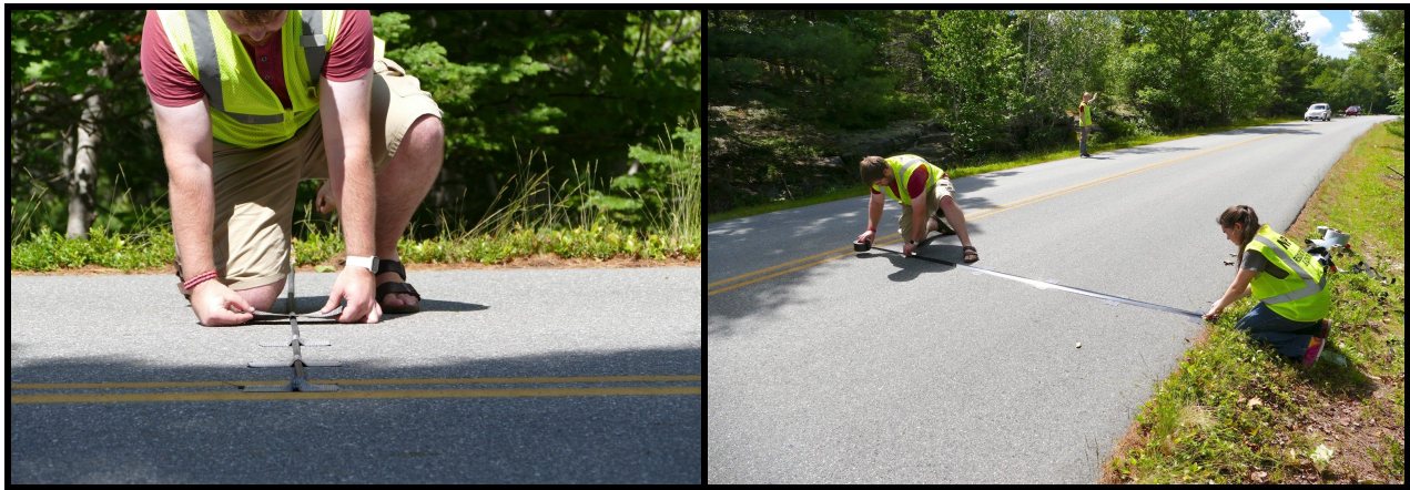
Figure 13: Installation of tube on Paradise Hill Road.
