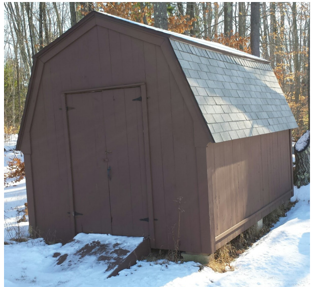
Figure 48: Shed Used for Testing
