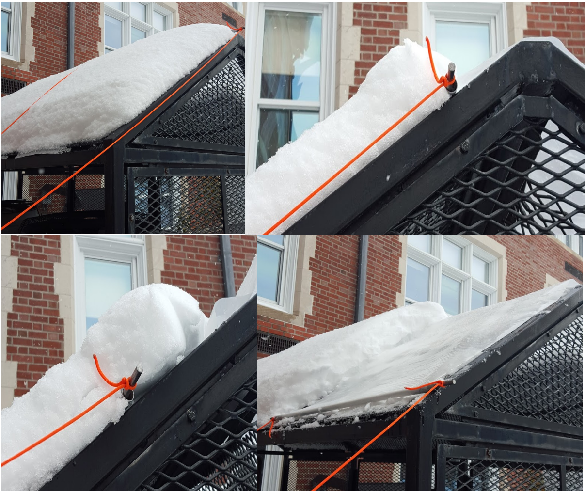
Figure 60: Tarp Roller Roof Clearing
