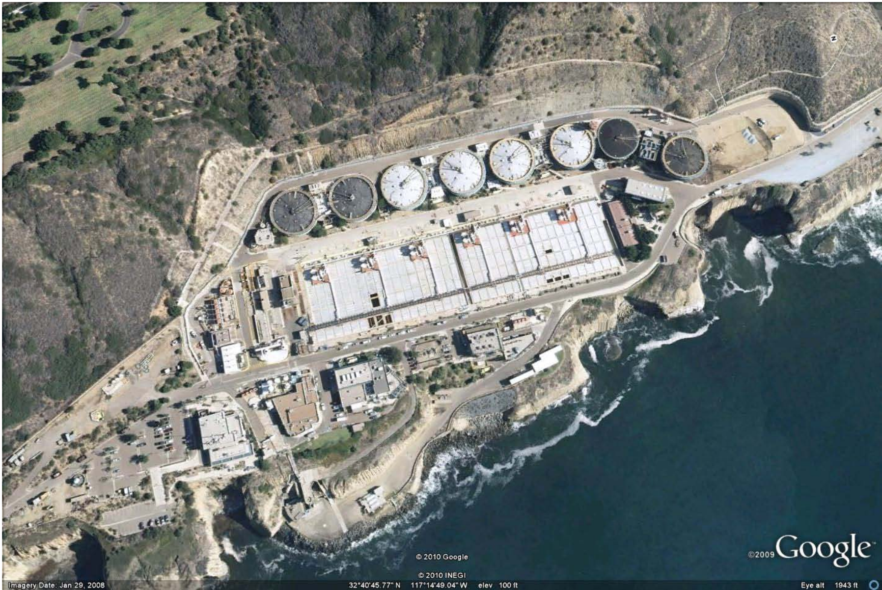
Figure 3-5: Aerial View of Point Loma Wastewater Treatment Plant in San Diego, CA (Source: Google Earth)
